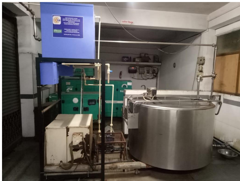
1 Heat Recovery unit Installed at Chuye BMC Center Gokul Dairy
